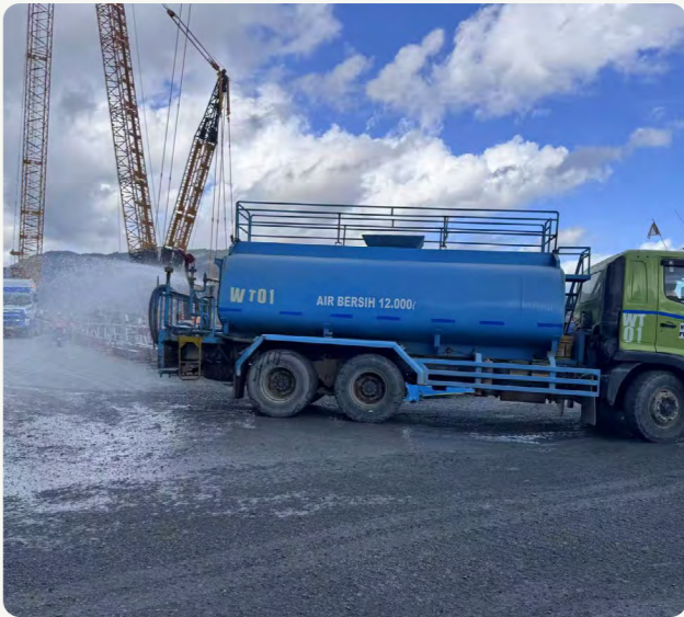
A water truck sprinkling water at the construction site to reduce dust 洒水车对施工现场进行洒水降尘
