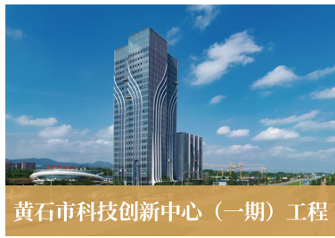
黄石市科技创新中心（一期）工程 Huangshi City Science and Technology Innovation Center (Phase I) Project
