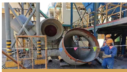
熔炼车间环保风机检修 Maintenance of environmental protection fan in meltshop
