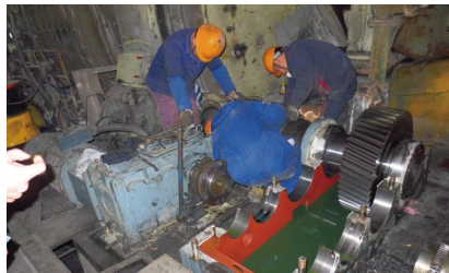
半自磨机减速机检修 Maintenance of semi-autogenous mill reducer
