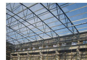
成品库钢屋架 Steel roof truss of finished product warehouse
