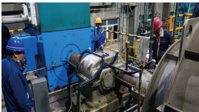
硫酸车间二氧化硫风机检修 Sulfur dioxide fan maintenance in sulfuric acid workshop
