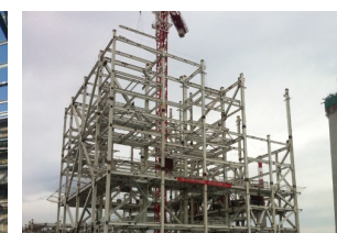
锅炉房 Boiler room
