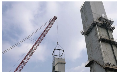
制氧空分塔检修 Oxygen air separator tower maintenance
