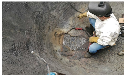
铜包焊接检修 Copper cladding welding maintenance
