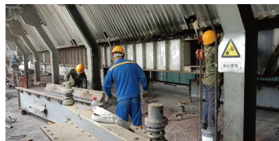
锅炉灰斗更换 Boiler ash hopper replacement
