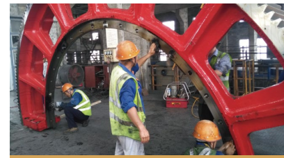
大修渣选4#球磨机大齿圈外观检查 Appearance inspection of big tooth ring for overhaul slag 4# ball mill
