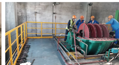
一期鼓风机房止推轴承维修 Maintenance of thrust bearing shell for air blower room (Phase I)
