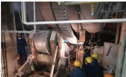
阳极炉托轮更换 Replacement of riding wheel for anode furnace
