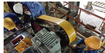
破碎机检修 Crusher maintenance
