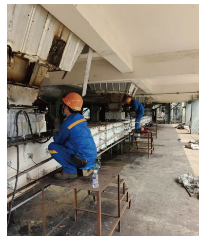
电收尘膨胀节更换 Expansion joint replacement of electric dust collector
