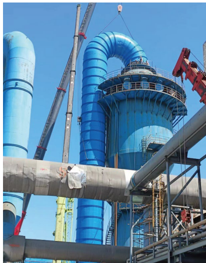
精炼车间洗涤塔出口管更换 Replacement of outlet pipe for scrubber in refining workshop
