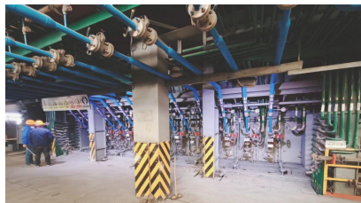
熔炼车间侧吹炉检修 Side-blown furnace maintenance in meltshop
